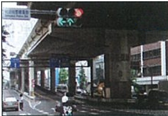
Metropolitan Expressway (Tokyo, Japan)
