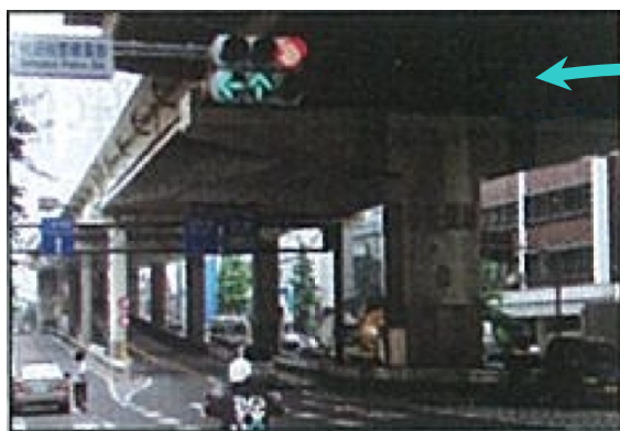
Structural health monitoring
