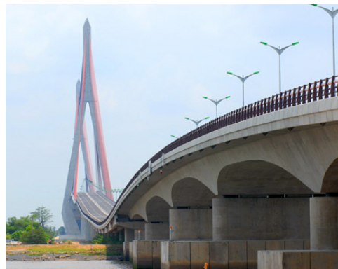
Can Tho Bridge (Vietnam)
