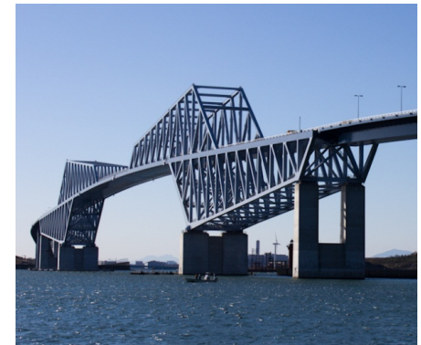
Tokyo Gate Bridge (Tokyo, Japan)
